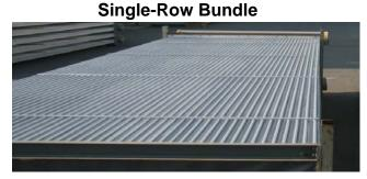
Primary – Main condensing, concurrent flow between steam and condensate Secondary - Non-condensable gas venting and condensing, Countercurrent flow
