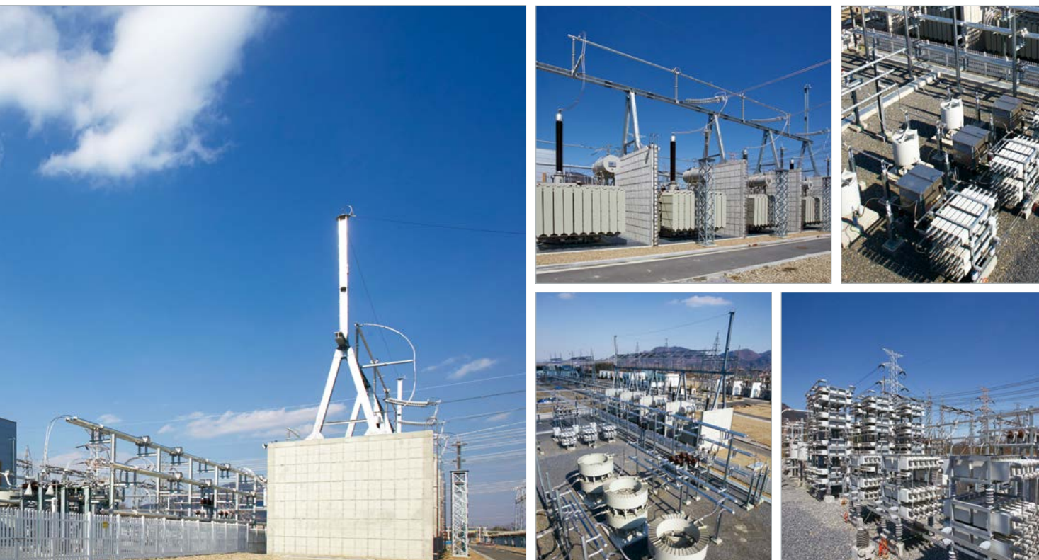
SVC Substation, Korea | The largest capacity in a single SVC Substation, rated at -225/+675 Mvar
