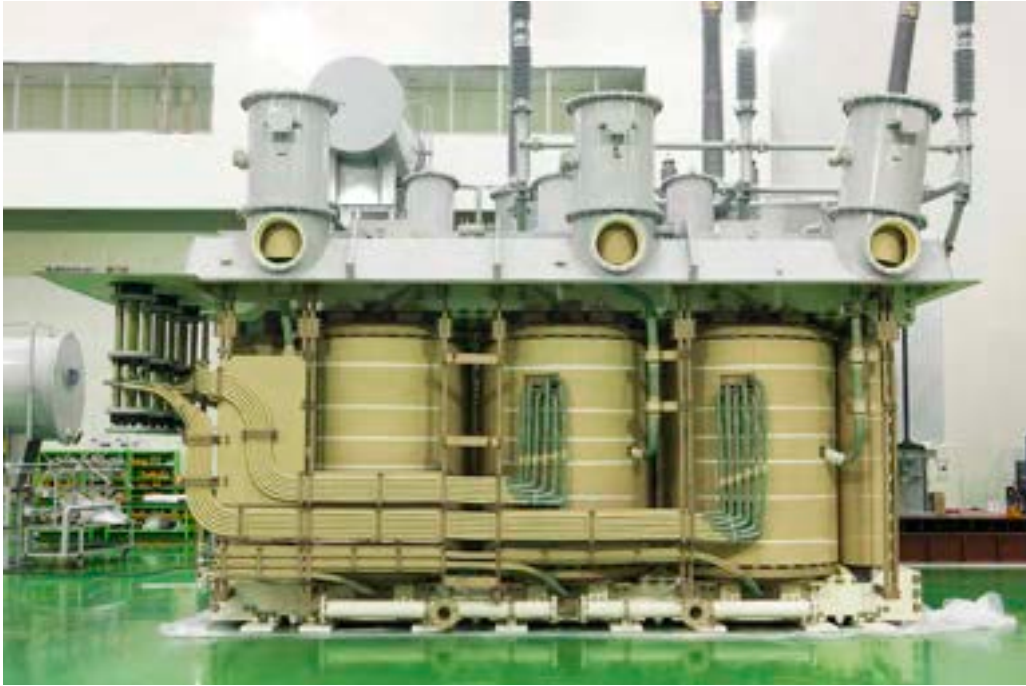
· CORE AND COIL ASSEMBLY
