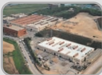
• Hwaseong 1 st Plant
