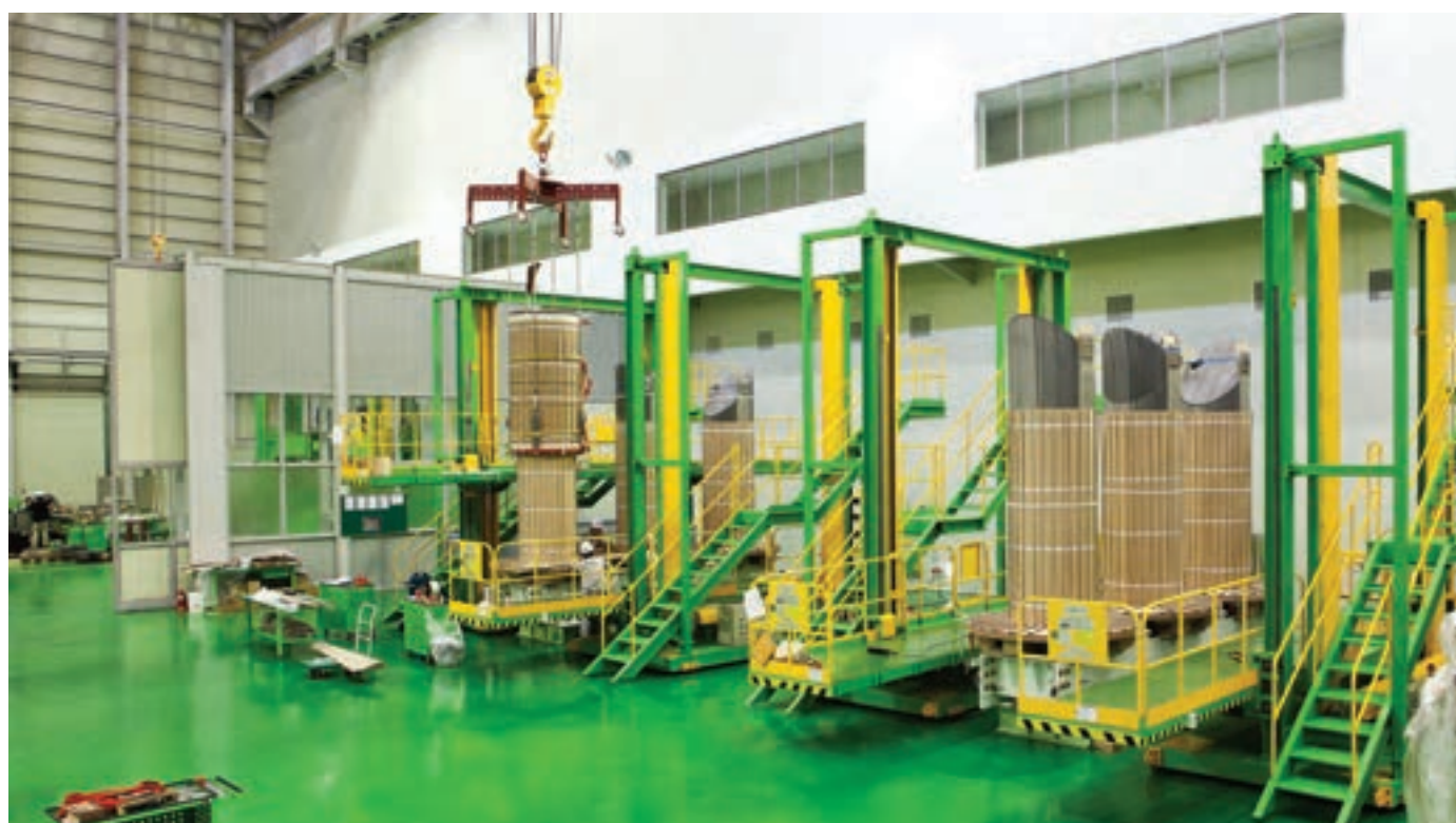
· CORE AND COIL ASSEMBLY SHOP
