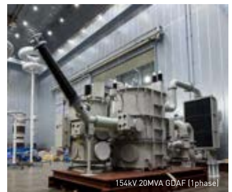
154kV 20MVA GDAF [1phase]
