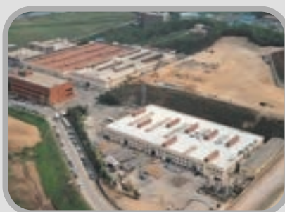
• Hwaseong 1 st Plant
