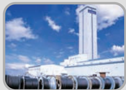
• Hwaseong 2 nd Plant
