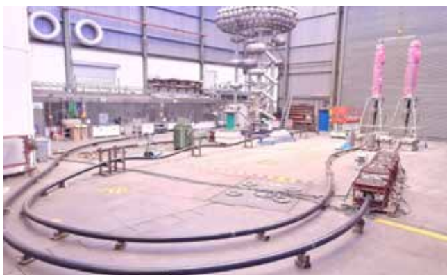
[ ±320kV VSC type XLPE cable system PQ test loop at KEMA FGH ]
