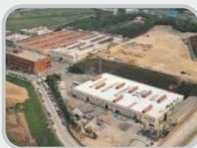
• Hwaseong 1 st Plant
