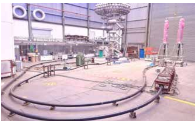
[ ±320kV VSC type XLPE cable system PQ test loop at KEMA FGH ]
